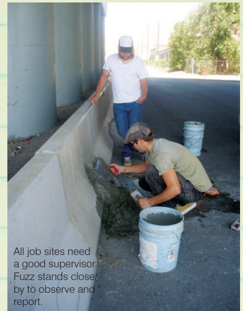
Bberex uses his professional skills and concrete trowels to bevel the ends of the transition. Beveling will help prevent crumbling.
