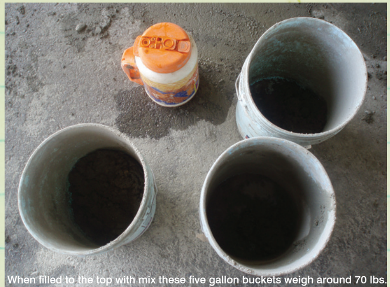
When filled to the top with mix these five gallon buckets weigh around 70 lbs.
